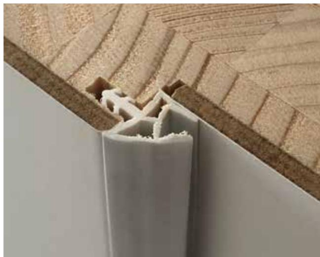
The aesthetic simplicity of the FEEL line merges with the need for privacy and comfort inside the home. The doors achieve acoustic insulation performance ranging from 22 dB in the standard version up to 41 dB in the certified version, thanks to their solid structure and special gaskets. Furthermore, the softness of the gaskets and the magnetic lock ensure silent opening and closing phases.
